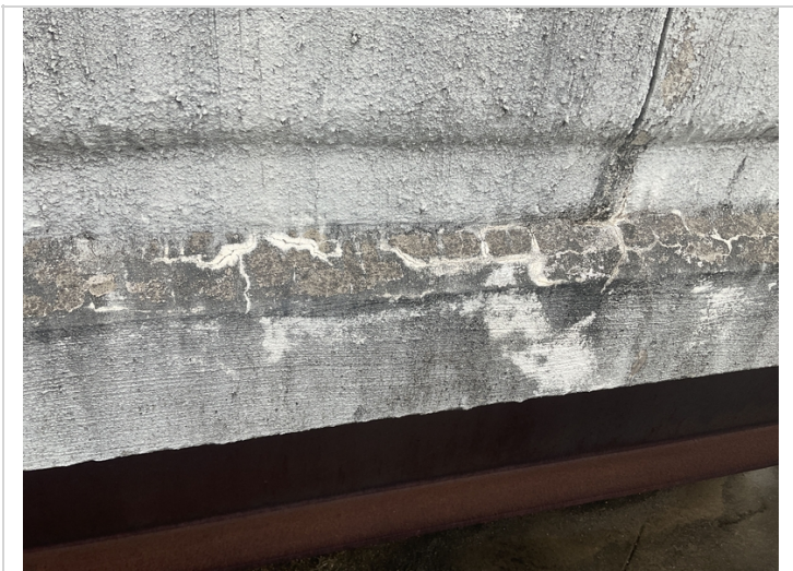
Efflorescence in concrete bridge railing various locations
