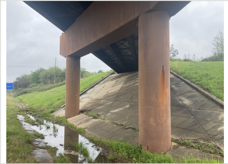
Rust staining on all 6 Columns
