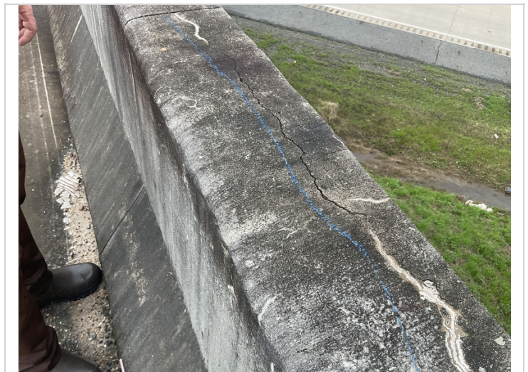
Cracking in concrete bridge railing various locations
