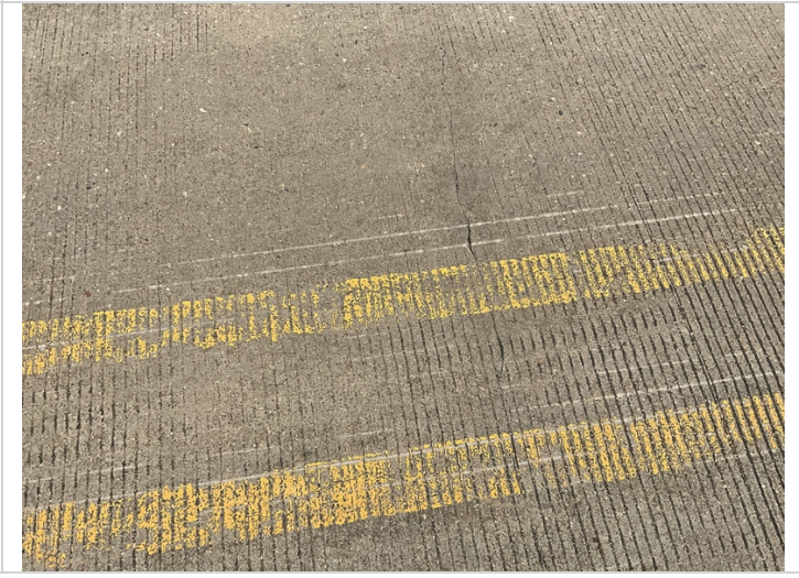
Cracking in deck various locations
