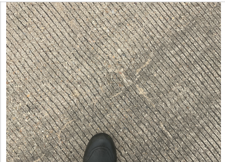
Cracking in deck
