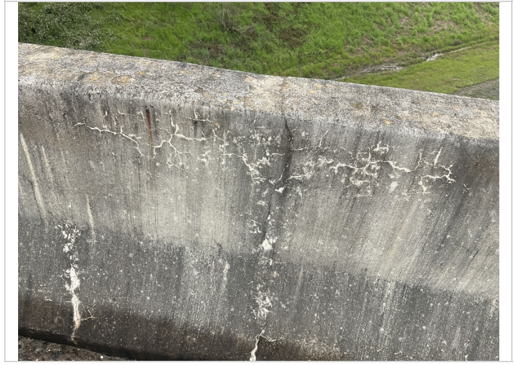
Map like efflorescence in concrete bridge railing various locations
