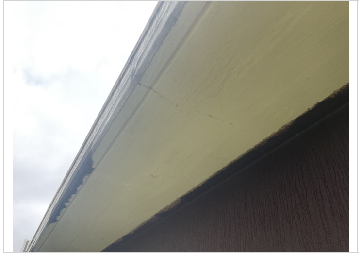
Cracking in deck overhang various locations
