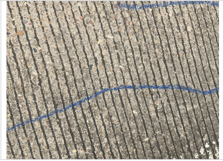
Minor cracking in deck various locations
