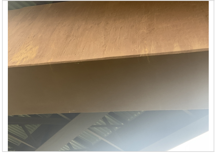
Small hairline cracking bent 3 cap
