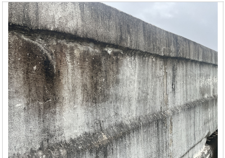
Cracking in bridge concrete railing various locations
